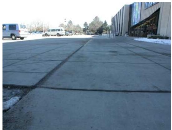
Figure 33 - Lip at End of Walk from Parking Garage
