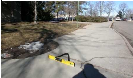
Figure 31 - Steep (4.9%) Cross Slope on Approach Walk new IMAX "After Hours" Entrance
