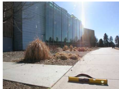
Figure 37 - Steep Cross Slope at Special Events Entrance Approach
