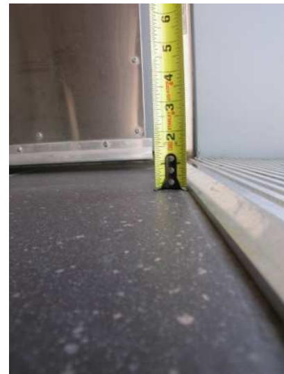
Figure 50 - Typical Inaccessible Metal Threshold Sky Terrace Restrooms
