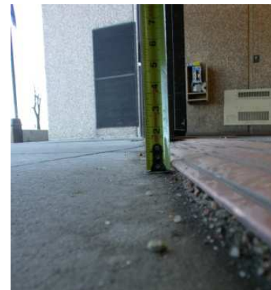
Figure 35 - High Threshold at the Eastern Most Main Entrance Doors
