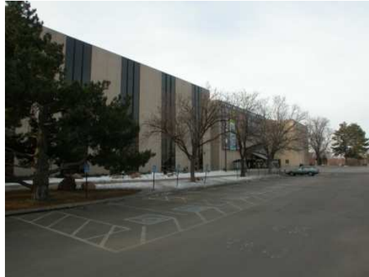
Figure 41 - Accessible Parking at Main Entry
