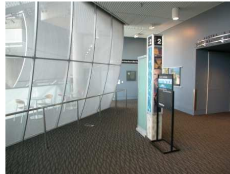
Figure 26 - Railing Not Cane Detectable on Level 2
