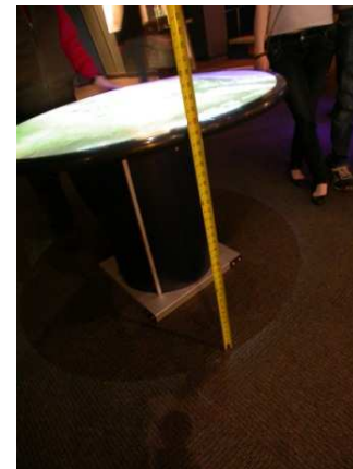
Figure 5 - Display Top Not Cane Detectable
