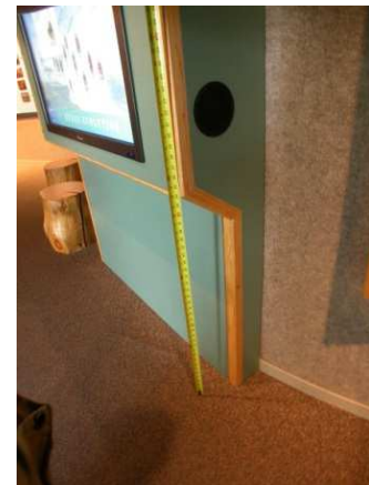
Figure 9 - Protruding Monitor
