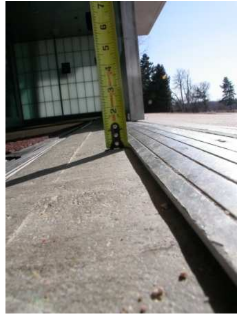
Figure 39 - High Threshold at Special Event Entrance
