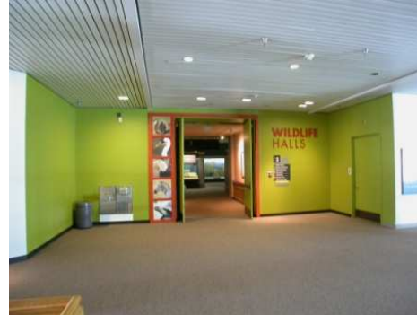
Figure 28 - Drinking Fountains Not Cane Detectable
