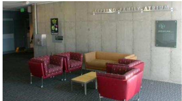
Figure 19 - Protruding Fire Extinguisher Box on Wall
