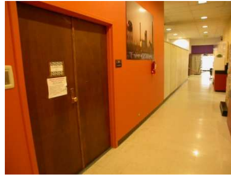
Figure 12 - Knob Hardware on Narrow Doors
