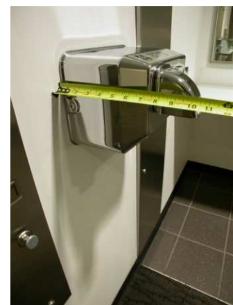
Figure 47 - Typical Protruding Hand Dryer
